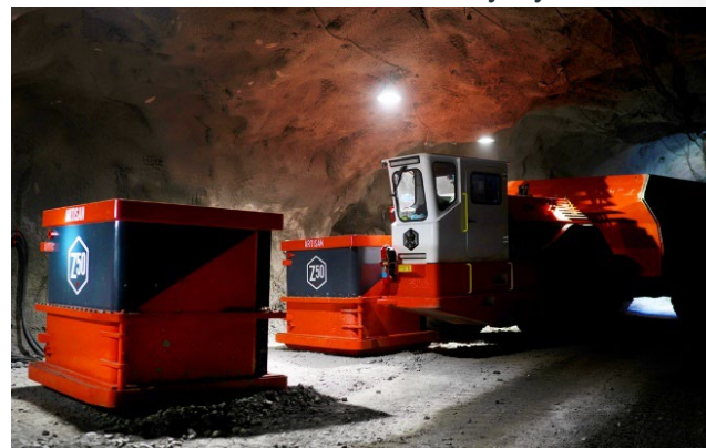
Artisan Battery Station
