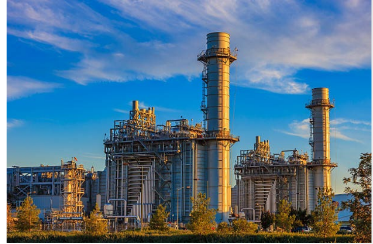
Natural Gas Power Plant
